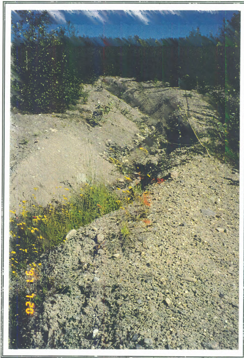
SITE SOV2. Deep gullying and erosion on an undeactivated road. The erosion occurred some time in the past and the site is stable now.
