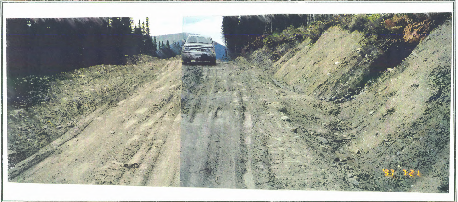
SITE M6. A recently constructed road in the upper McMartin Creek basin. Erosion of the road surface and the cut and fill slopes was very evident. No sediment control measures had been used.
