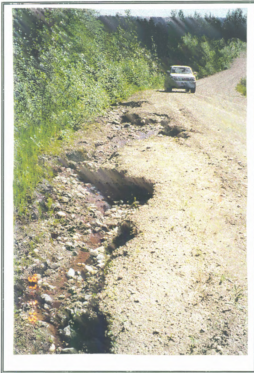
SITE U5. Road and ditch erosion in the Umiti Creek basin. The road itself is stable. However, the infrequent cross-drains allows surface runoff to concentrate and occasionally trigger extensive erosion. At this site, the ultimate discharge point was a tributary stream channel.
