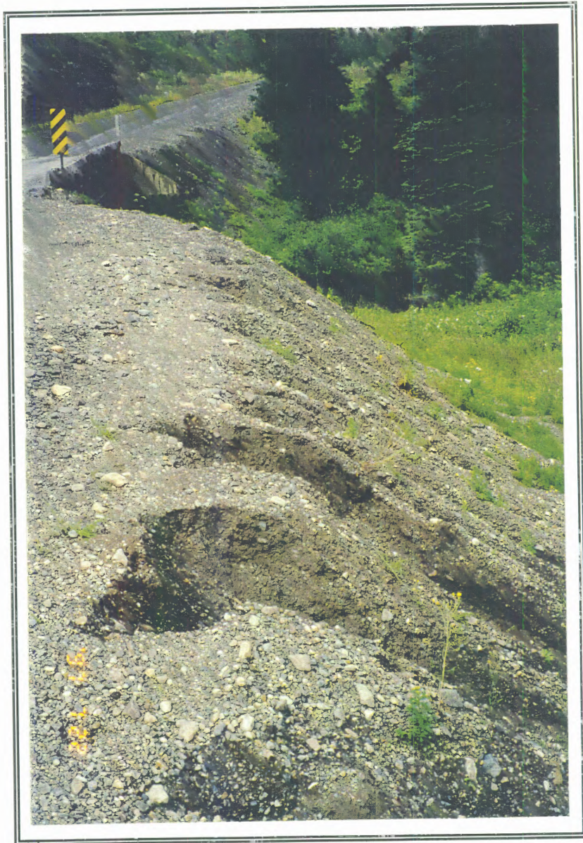
SITE V2. Erosion of fill material at a bridge crossing of Victoria Creek.
