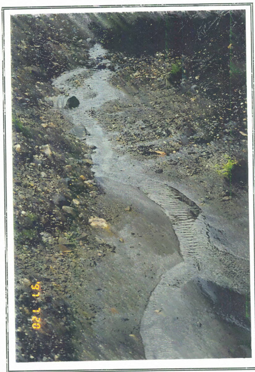
SITE LS8. An aggrading ditch line in the Little Swift basin. There is active erosion along the ditch and cut slope, and sediment is infilling the culvert.
