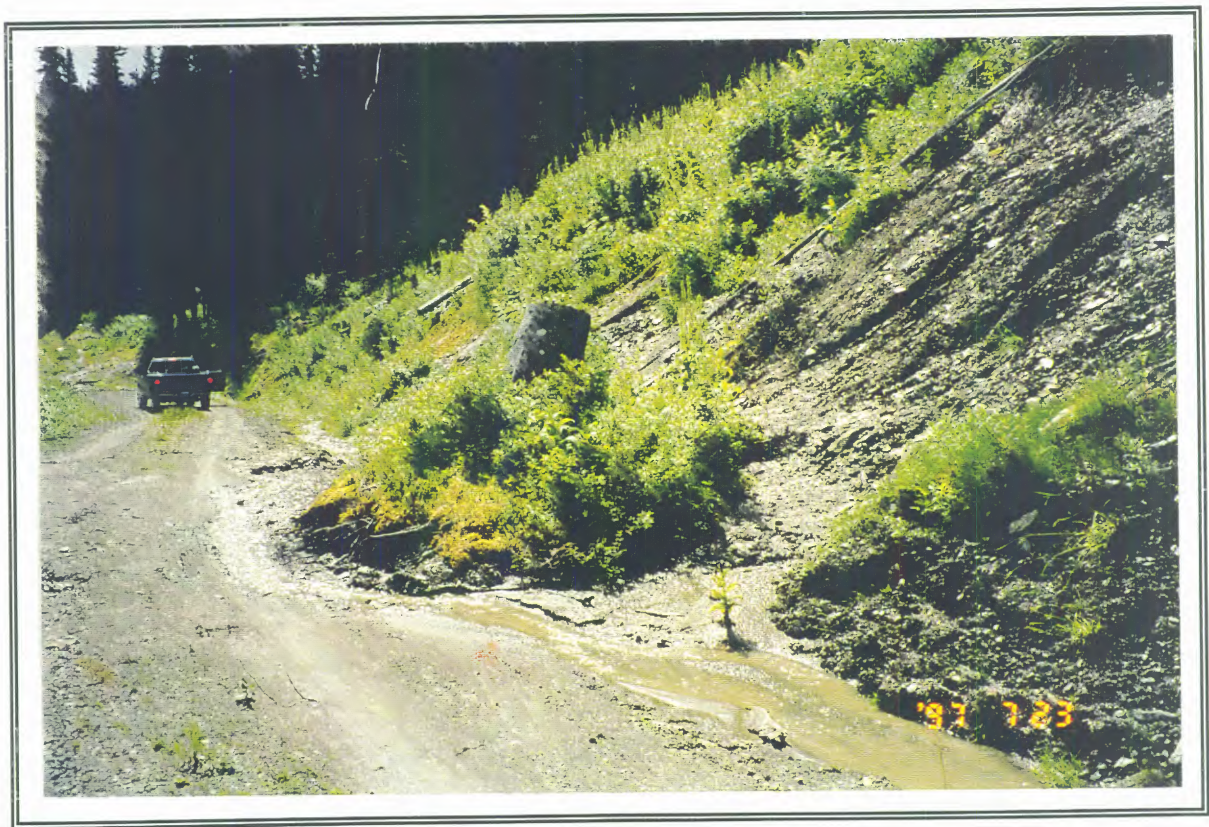
SITE L11. Cut slope slumping and ditch erosion in the xxx sub-basin of Lightning Creek. This piece of road needs increased cross-drain frequency to remove the runoff water from the ditch.
