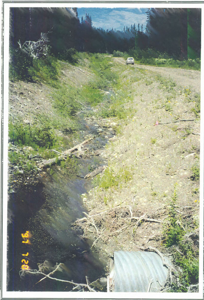
SITE R5. A ditch line in the Fontaine Creek sub-basin. Water is being concentrated in the ditch and some erosion is occurring.
