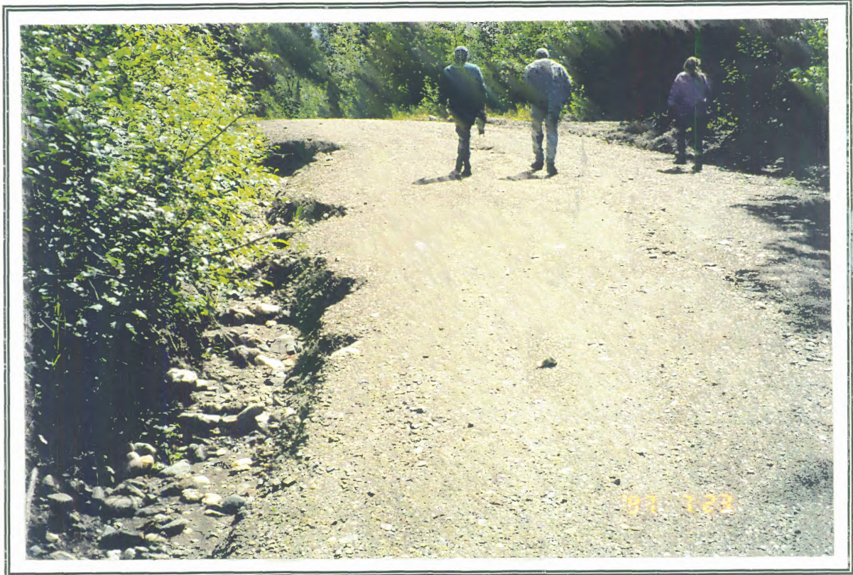
SITE L9. Ditch erosion along a mining road in the lower Lightning Creek watershed. This ditch discharges directly into Lightning Creek.
