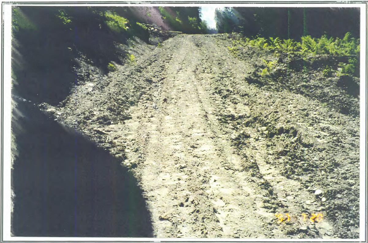
SITE R7A. A recently constructed road in the Fontaine Creek sub-basin. This site is experiencing extensive erosion. No sediment control measures have been used.
