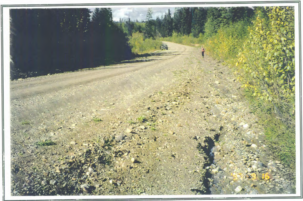
SITE JB6. Ditch erosion in the John Boyd Creek basin. This ditch drains about 150-200 m of road, and discharges directly into John Boyd Creek. The road itself is stable, but the ditch erosion transfers fine sediment into the creek.
