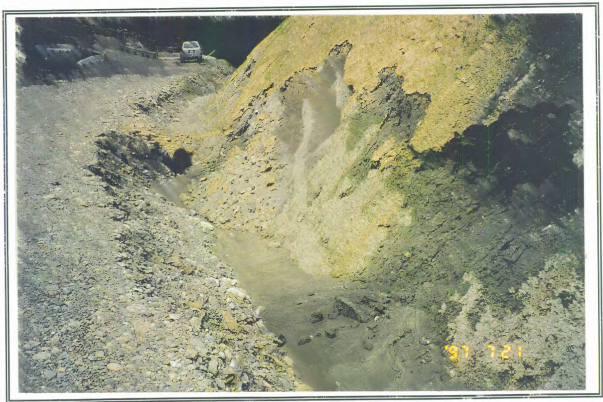
SITE M5A. Extensive cut slope erosion through a fluvial terrace. An attempt has been made to deal with this erosion by grass seeding the sandy cut slope. However, this has failed and the slope is continuing to slough large amounts of sand-sized material into the ditch. This sediment enters a tributary to McMartin Creek.
