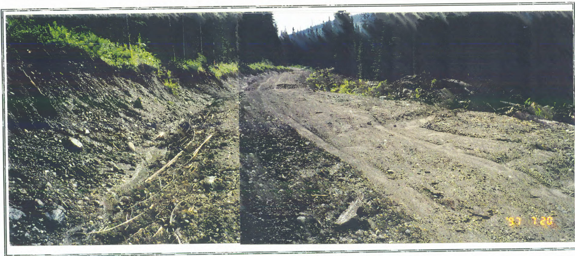
SITE LS6. A recently constructed road in the upper Little Swift River basin. The site disturbance and lack of erosion control has resulted in large amounts of fine sediment being transferred to a tributary stream.
