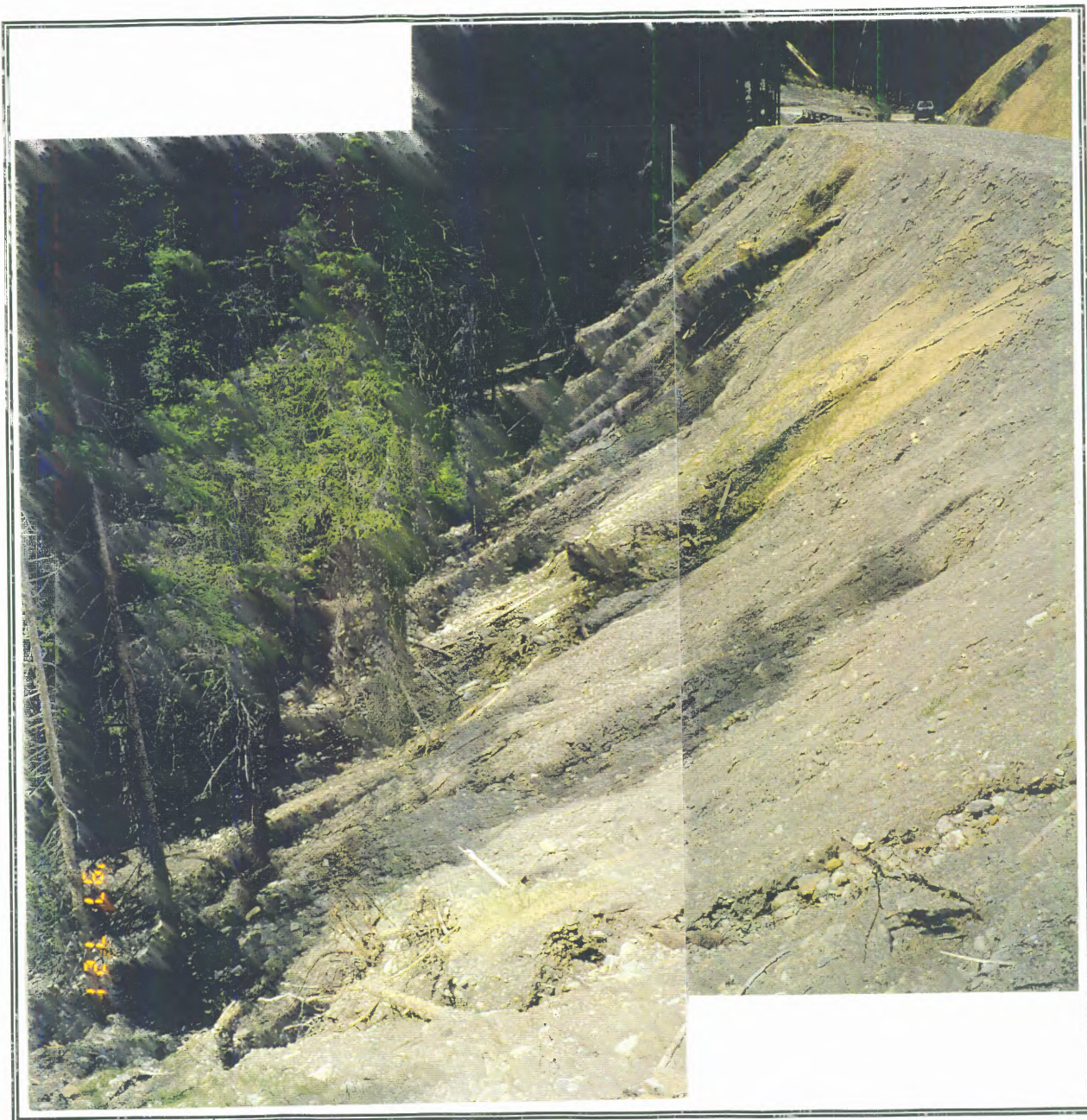
SITE M5B. The road fill is fine textured, and is not stable. An attempt has been made to control erosion by applying grass seed, but this has not succeeded. This slope is supplying large amounts of fine sediment to a tributary of McMartin Creek.
