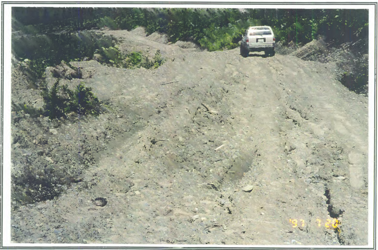
SITE R7B. A recently constructed road in the Fontaine Creek sub-basin. This site is experiencing extensive erosion. Note the rutting and the eroding running surface and cut slope.
