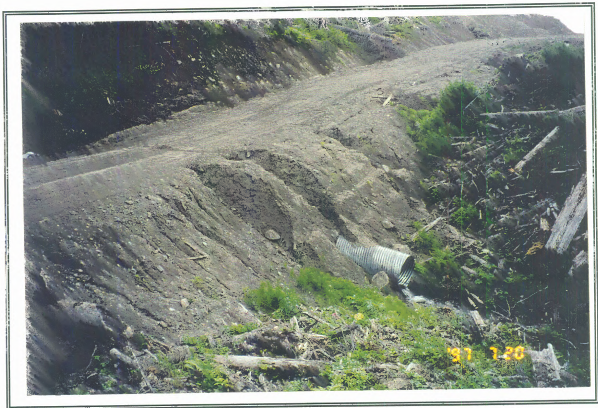
SITE LS7. A recently constructed road in the upper Little Swift River basin. At this site the fine-textured road fill is being eroded by water flowing along the road surface and ditch. The eroded sediment discharges directly into a tributary to the Little Swift River.
