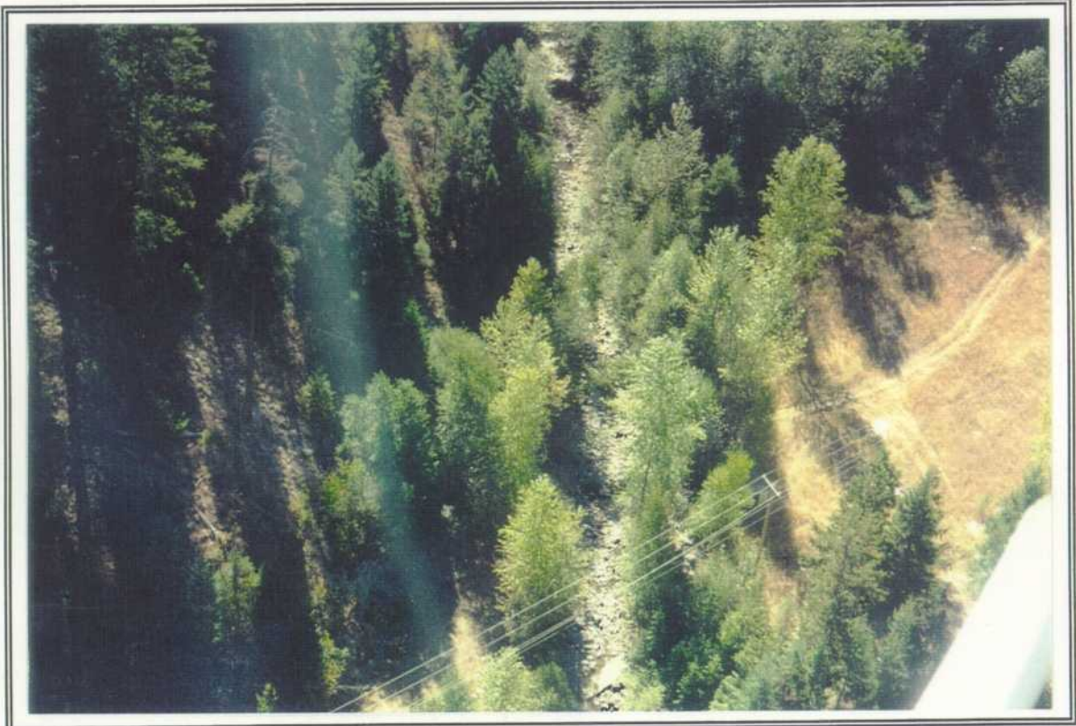
PHOTO KA-2. Reach KA - Overview (RA4, P15)
