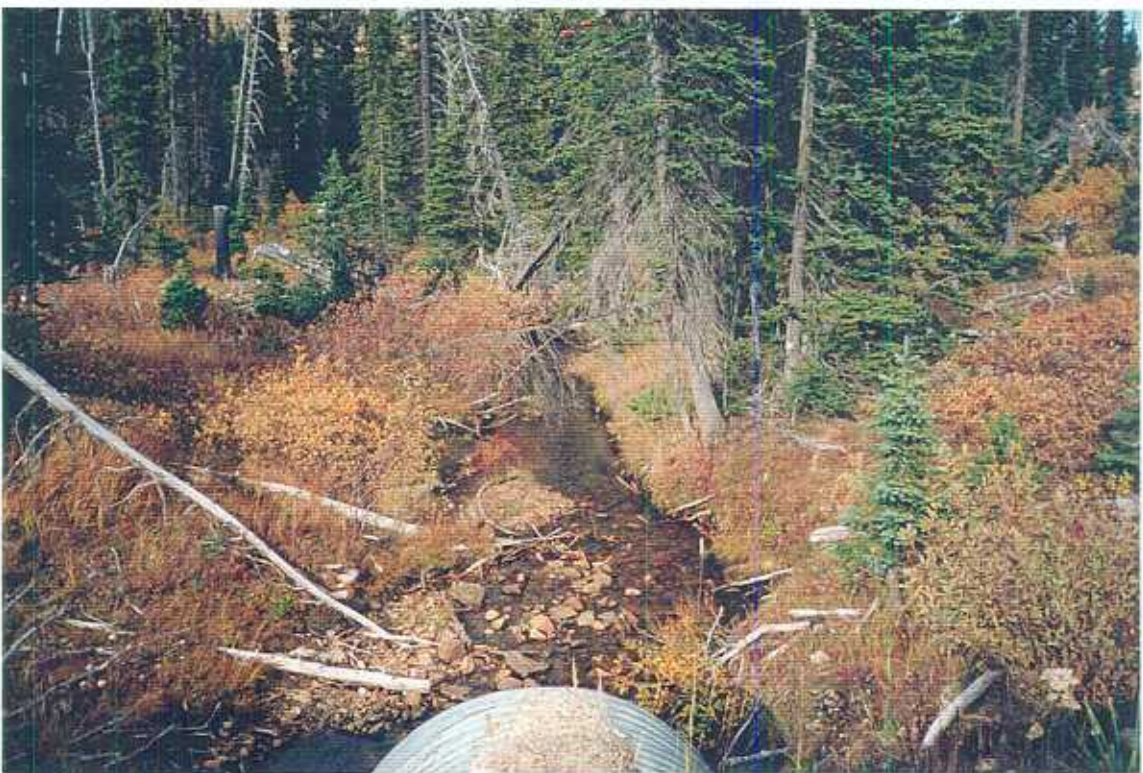
Photo 70: Granite Creek. View of Site 4 facing downstream. Note undercut banks. (6 October 1996).
