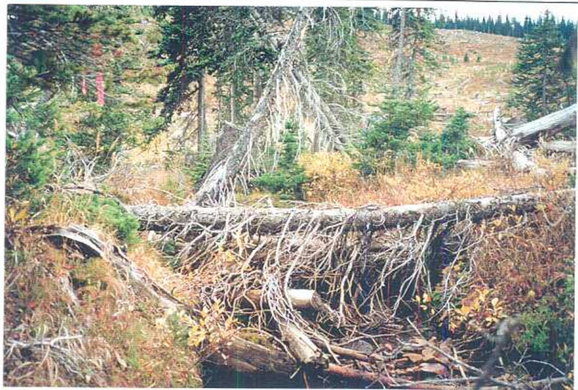
Photo 75: Granite Creek. View of Site 4 downstream of culvert facing upstream. Note pool completely under bank and debris in stream. (6 October 1996).
