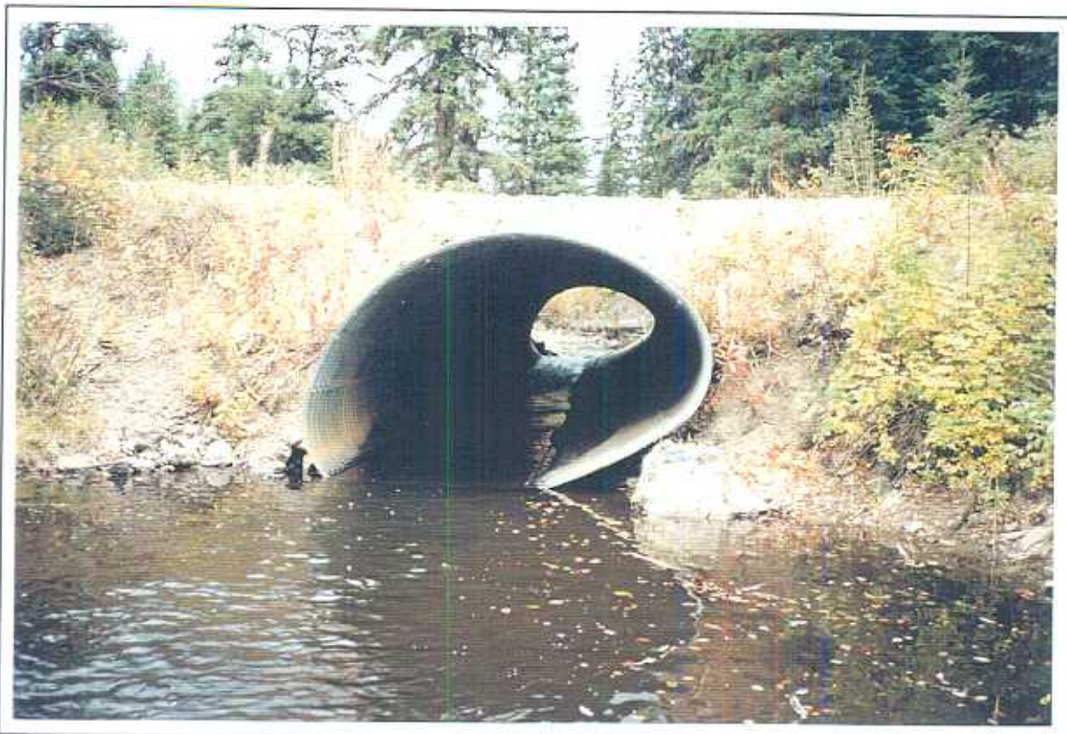
Photo 115: Otter Creek. View of Site 5 facing upstream through culvert. (3 October 1996).
