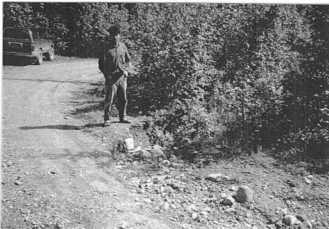
Photo 2. Erosion of the road surface adjacent to the d/s end of the culvert, d/s view. Stream Name: Brash Creek Site #: 12 Reach #: 2 Coordinates: 49°45.10' 119°20.20' Code: Fs/Q•C•F•1
