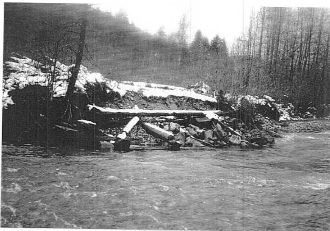
Photo 2. Wap Creek: Washed out bridge abutments at Site #4.
