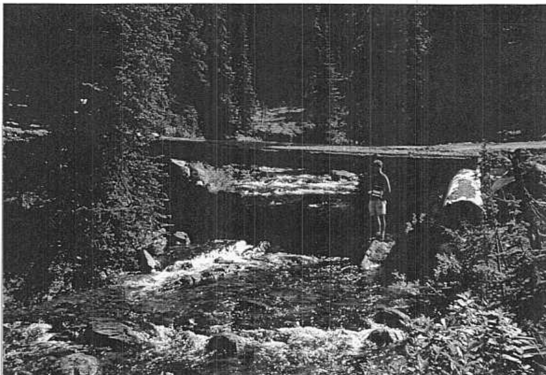
Photo 2. Steel-span (railway cars) bridge with rotting wood deck and erosion of road surface, u/s view.
