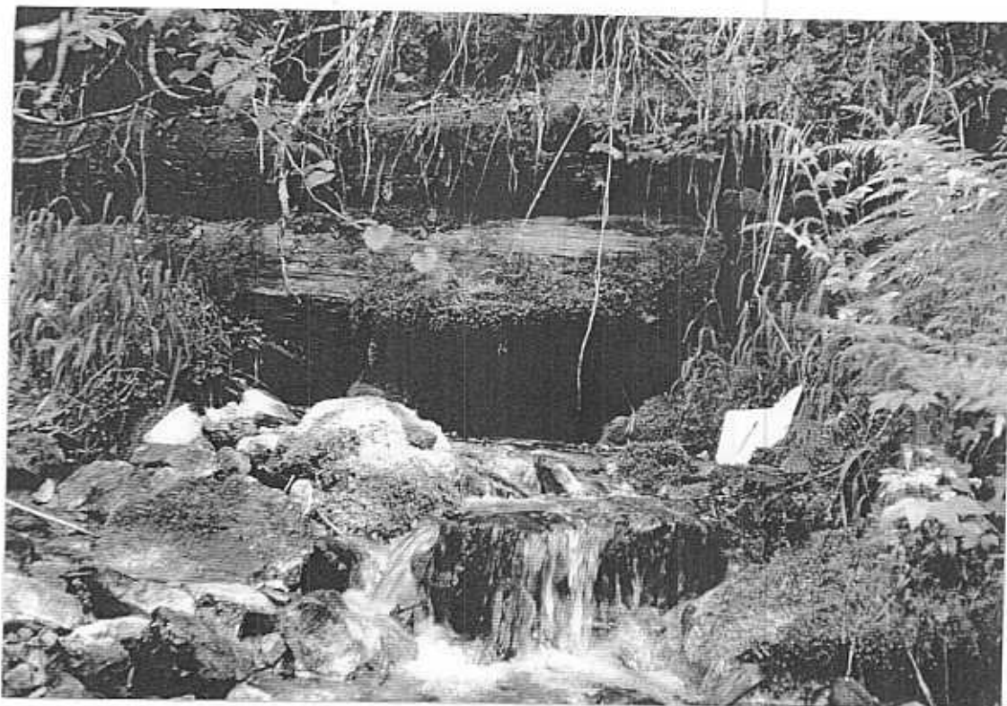
Photo 3. Culvert outlet with overlaying logs and restrictions on stream width and peak flow, u/s view. Stream Name: Brash Creek Site #: 13 Reach #: 2 Coordinates: 49°45.23' 119°20.19' Code: Fs/Q•C•F•1
