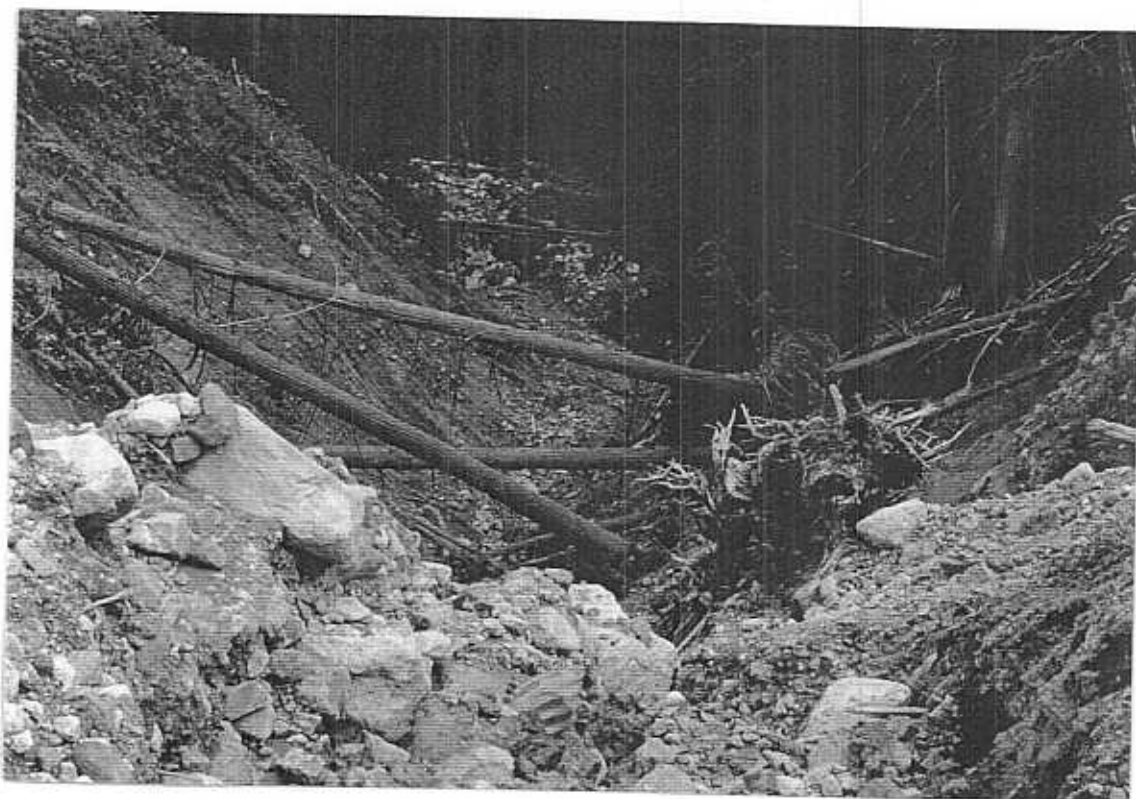
Photo 2. Landslide track looking downslope towards Hound Creek. Note culvert remanants in the foreground.
