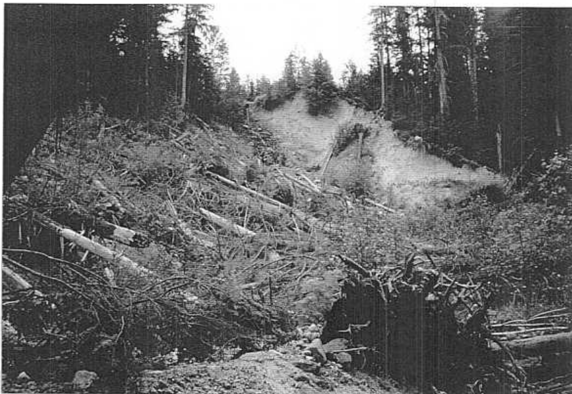
Photo 1. Debris and exposed bank associated with the slide at the culvert outlet, view from base of slide. Stream Name: Cooke Creek Site #: 8 Reach #: 2 Coordinates: 49°45.23' 119°20.19' Code: Fb/Fs/Q•C•F•1
