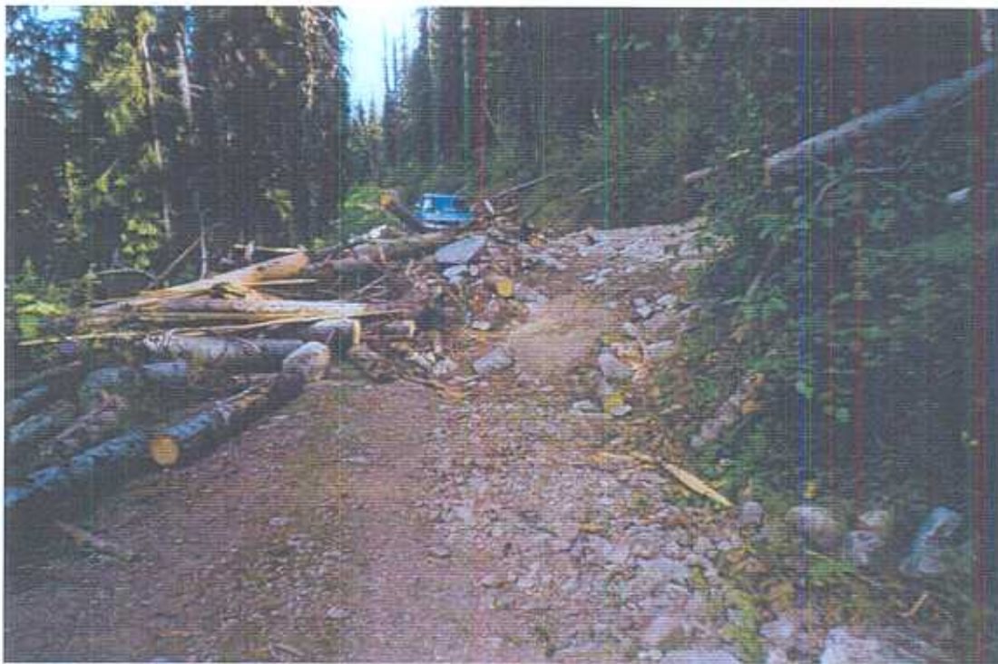
Plate 13: Debris flow (S15) track crosses the Sitkum Creek FSR at 11.5 km, resulting in 4x4 passage.
