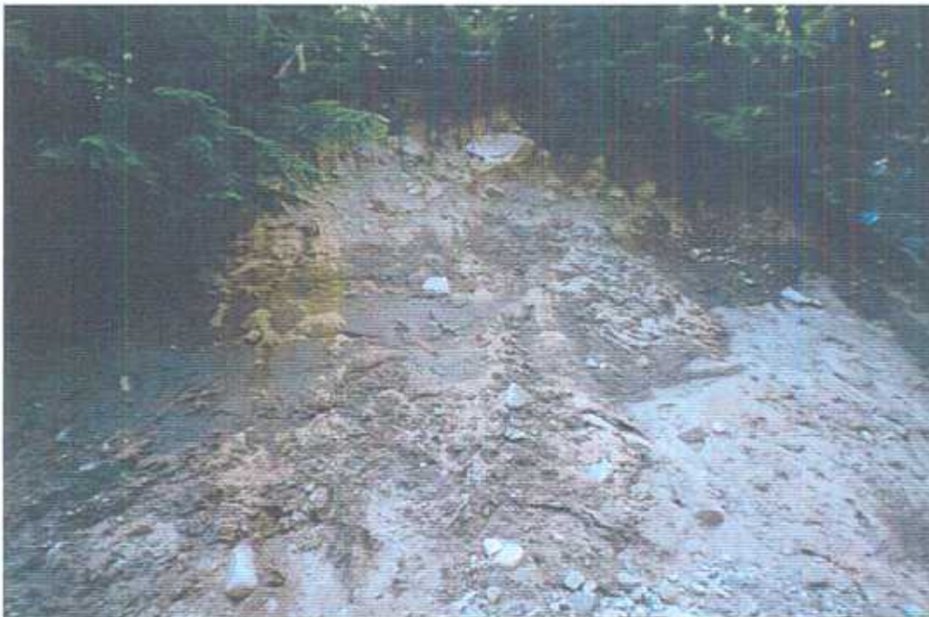
Plate 10: Road cutslope approximately 200 m upgrade of the Sitkum Creek road crossing. The seepage zone between sandy till and fine-grained glaciofluvial deposits is evident.
