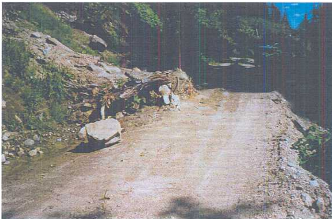
Plate 12: Cutslope slump at 8.13 km along Sitkum Creek FSR. Marked with stake as "#1" in the field. Date: 02-Aug-2000 Photograph 4-8
