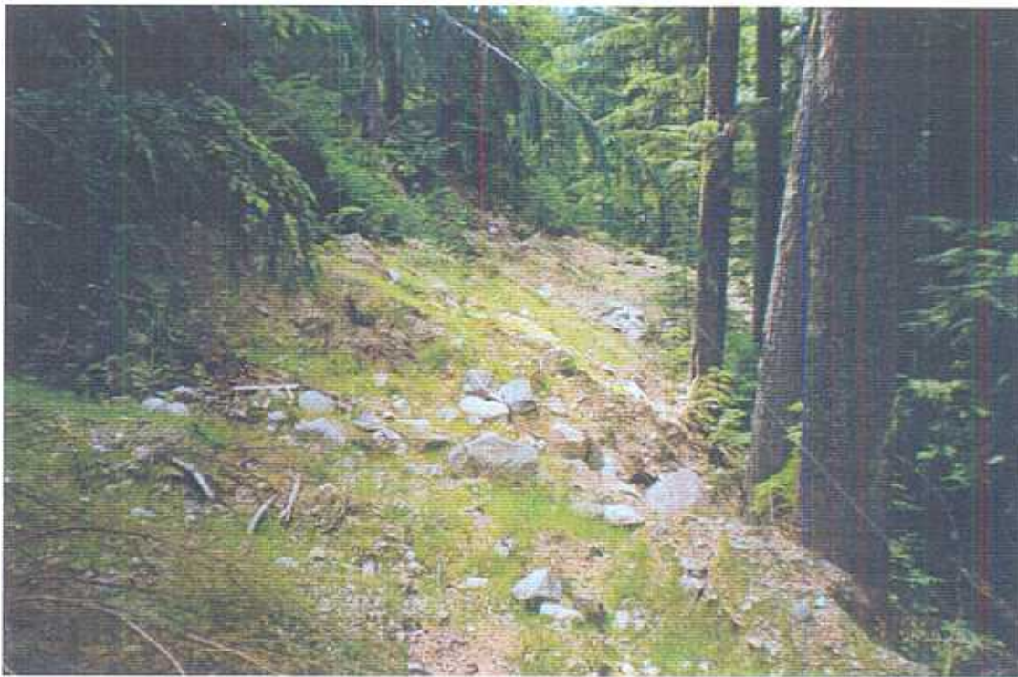
Plate 15: Typical view of Old Sitkum Creek road, with full pullback deactivation. Date: 03-Aug-2000 Photograph 4-32
