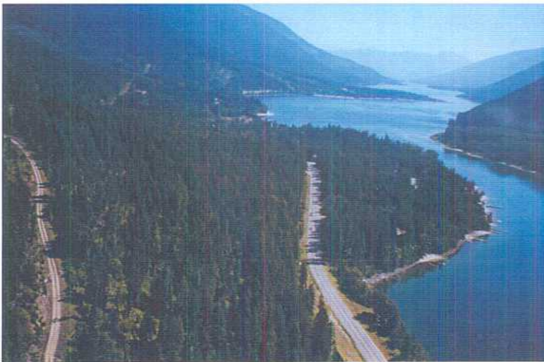
Plate 2: View east towards the Sitkum Creek fan at Kootenay Lake. Highway 3A crosses the fan and the Sitkum Face Road is at left. Date: 02-Aug-2000 Photograph 3-22
