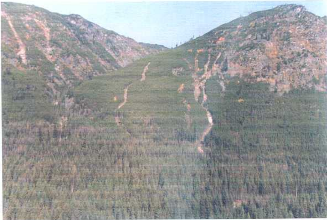
Figure 2. Erosion on a hillside along Raft River Road 9.
