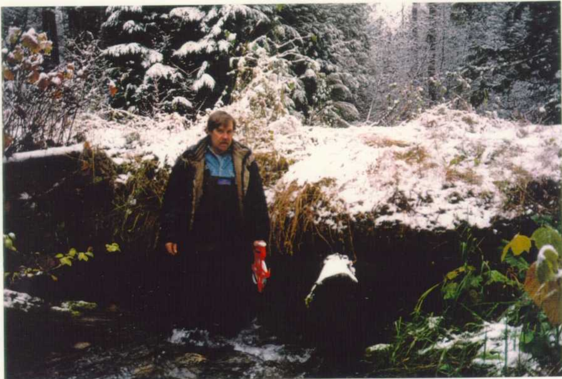
The bridge at site 2604 should be replaced since it provides access to private property (Fiddlestick campground).
