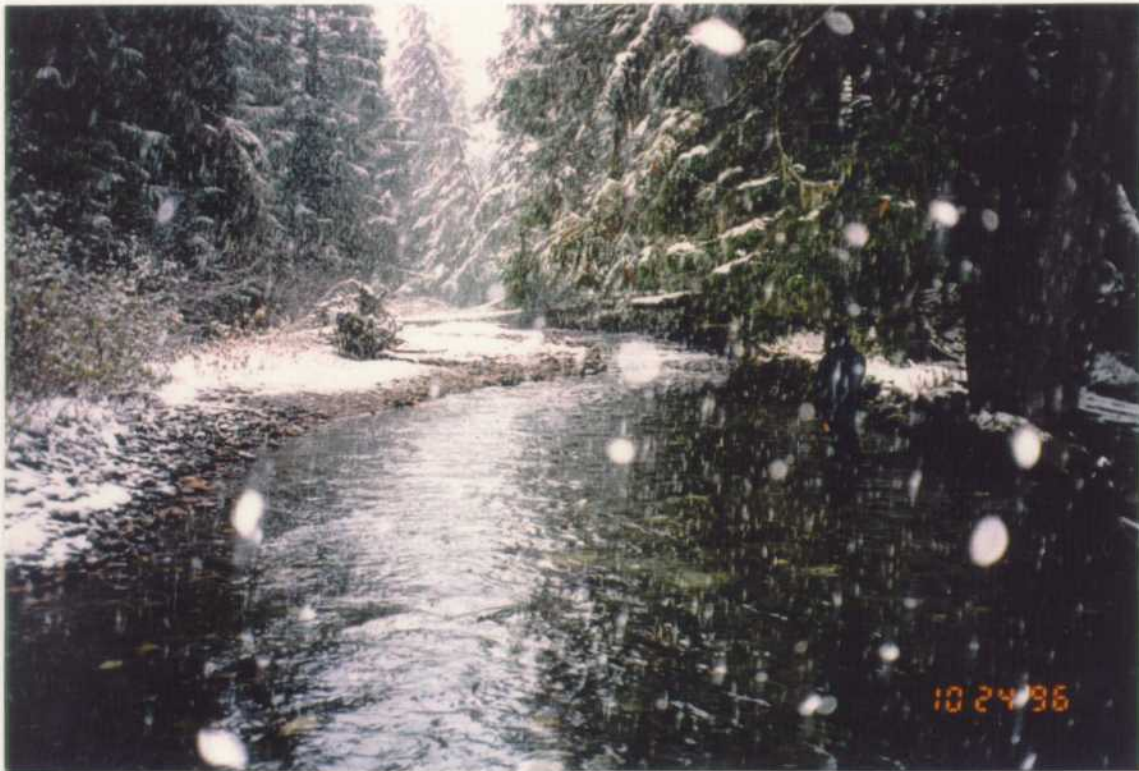
Downstream of the bridge. Upstream view of Reach 6B shows extensive riffle, sediment fingers and wedges and disturbed stonelines in this heavily aggraded channel.
