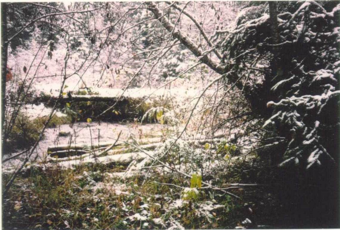
The side channel in the foreground and the old bridge in the background are features of site 2604.
