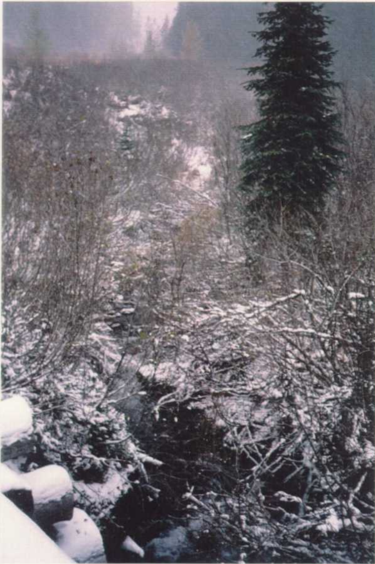
Downstream view of Reach 2, Pinnacle Creek shows the bridge crossing over a stable channel.
