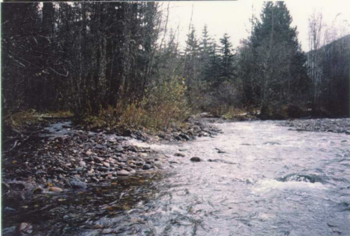
Upstream view shows multiple channels, potential off-channel habitat and aggradation.
