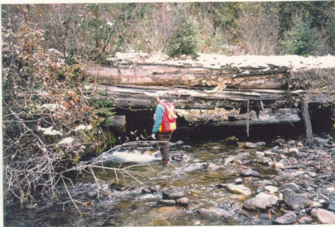
The bridge has vegetation growing on it, rotten stringers, 3 of 4 abutments are eroded, the bridge is sinking and sediment is evident in the channel. The bridge requires removal.
