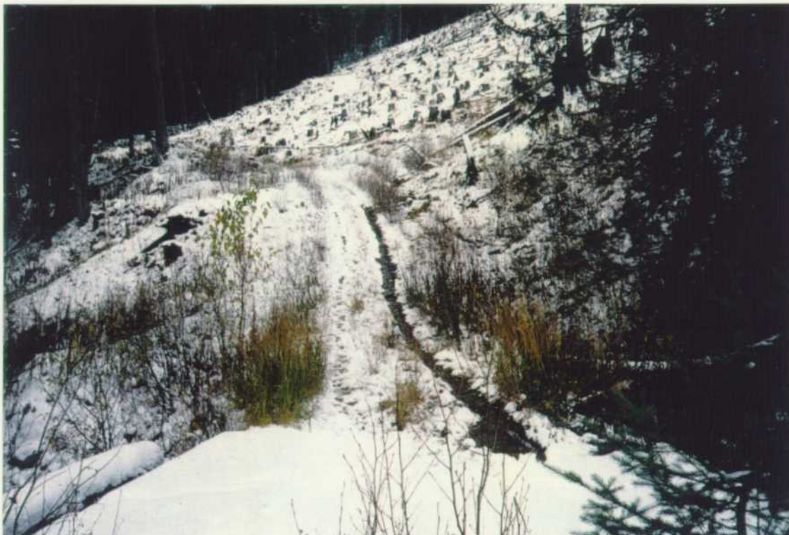
Water is running down the road, settling on the bridge and overflowing into the creek, therefore the drainage needs to be improved.
