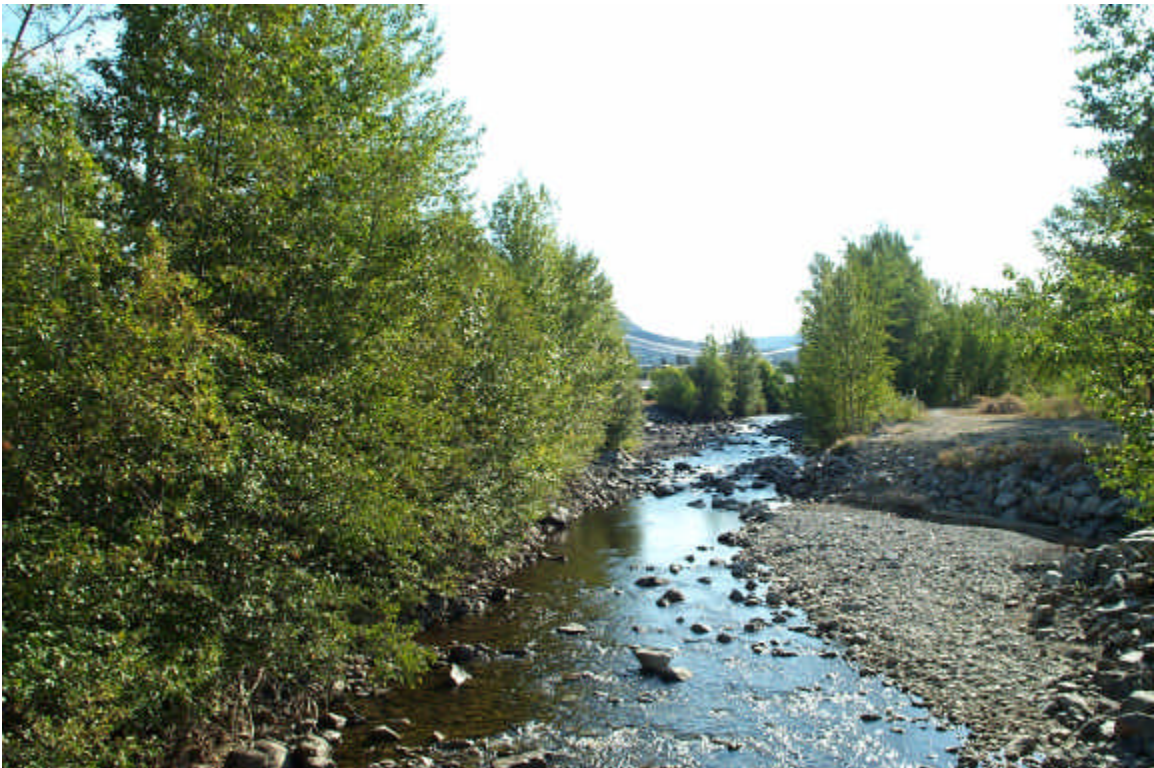
Photo 6. Looking upstream at demonstration riffle constructed in Mission Creek on August 29, 2000.
