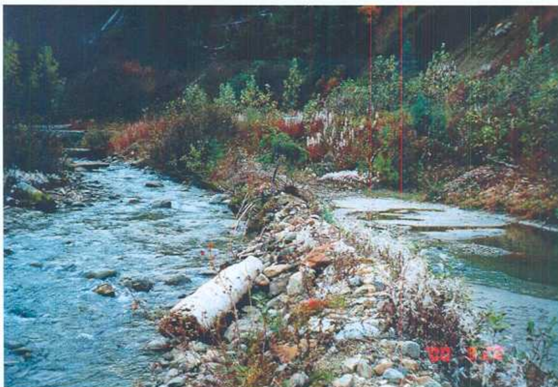
Photo 38: East Fork of Manteau (reach 1) – Berm constructed to protect road prism adjacent to bridge on Road 1211.
