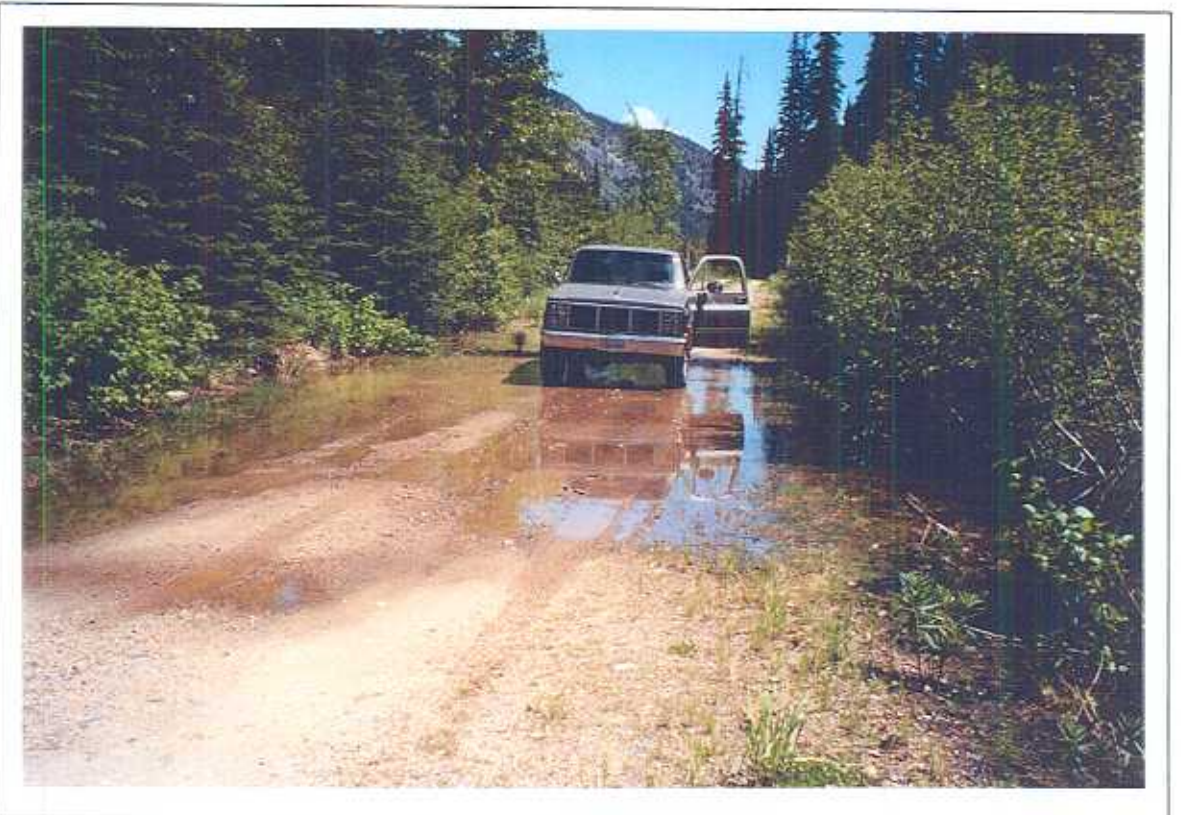
Photo 19: Culvert recommended at SS5 to prevent flow over road.
