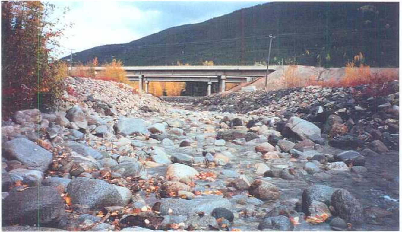
Photo 1: Juliet below confluence with July Creek. Note armoured banks upstream and downstream of Coquihalla highway.
