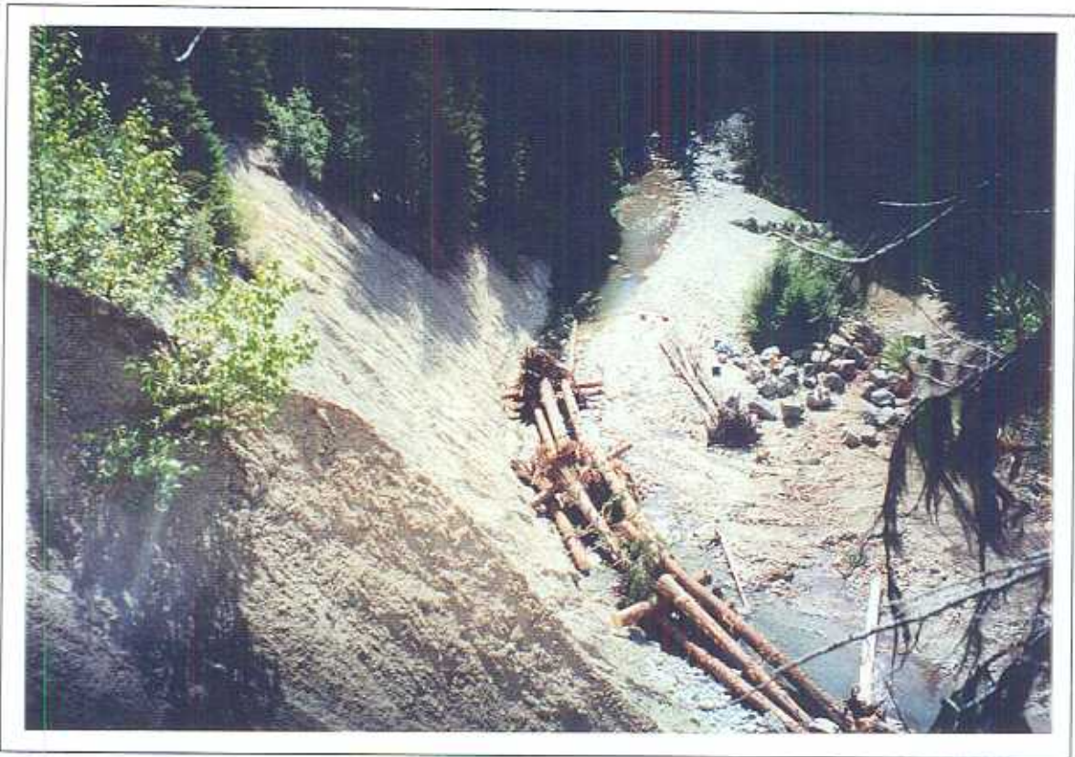
Photo 16: MW1, with slope stabilization works in progress.
