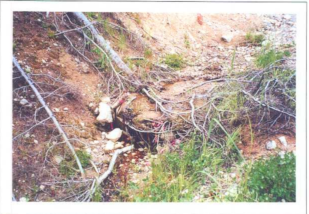
Photo 21: Full sediment silt fence at SS9.
