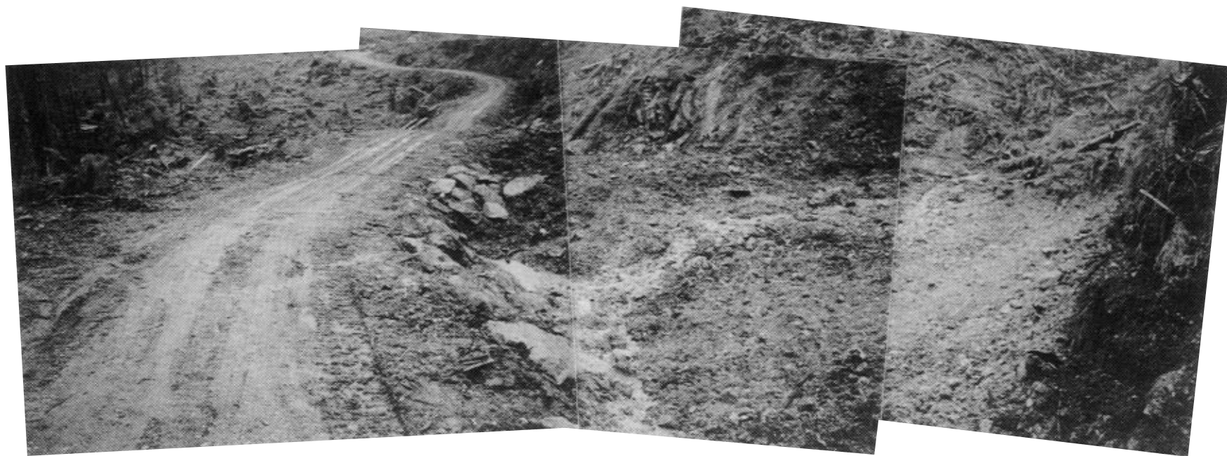
Road on left forms terminal berm for small debris basin. Note armouring on upslope side of road.
