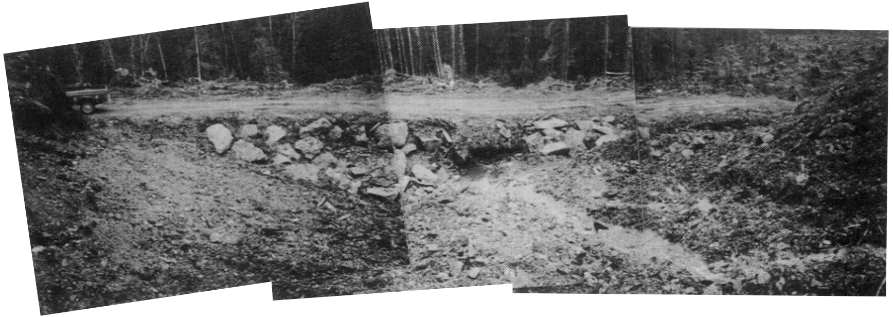
Looking downstream towards terminal berm. Note armouring.
