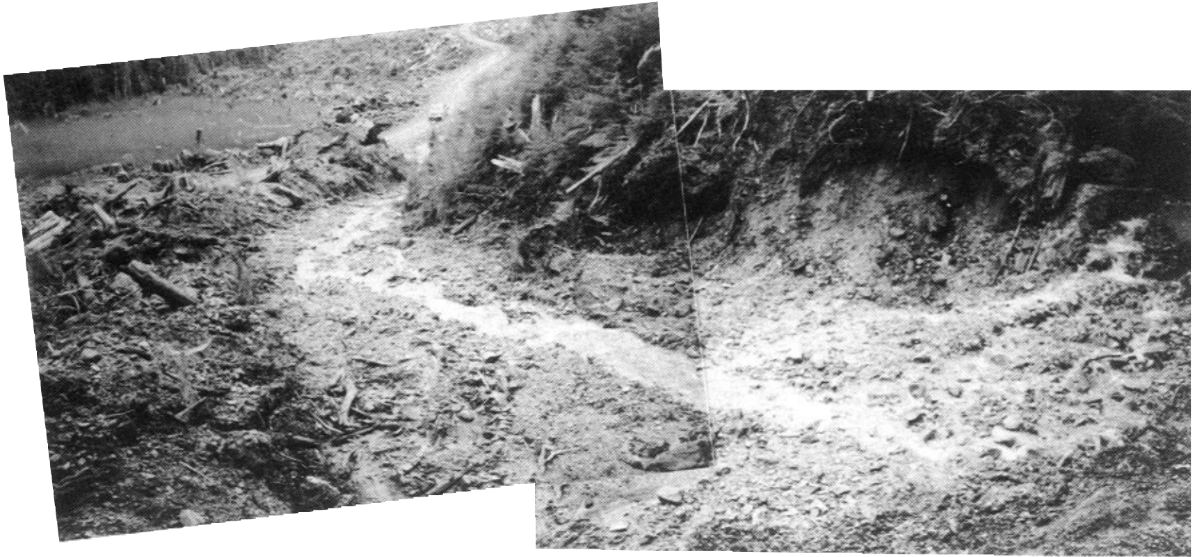
Looking downstream. Deflection berm is on left. Upslope side of berm has not yet been armoured.
