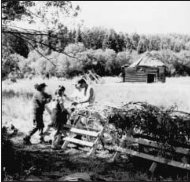
Figure 5. Student technicians from Saik'uz First Nation prepare willow wattles for bank stabilization.
