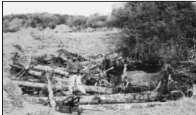
Figure 4. The site of a LWD root revetment during construction.
