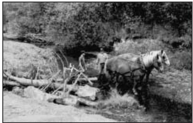
Figure 2. Nechako Valley Horse Logging's draft horses place large woody debris and boulder structures in Corkscrew Creek with precision and little environmental disturbance.
