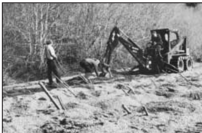
Figure 8. Machine planting in 1999, using large (1m and larger) willow and cottonwood cuttings.
