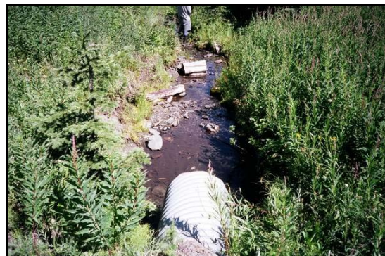
Photograph 8 – Site 32 Outlet Downstream View (Roll 6 Photo 3)
