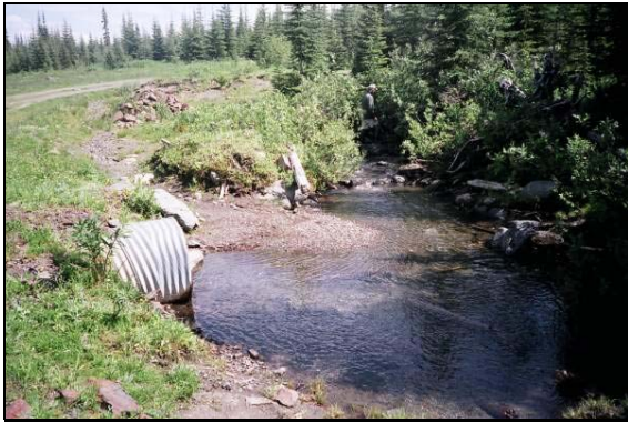
Photograph 1 – Site 13 Inlet Upstream View (Roll 1:9)
