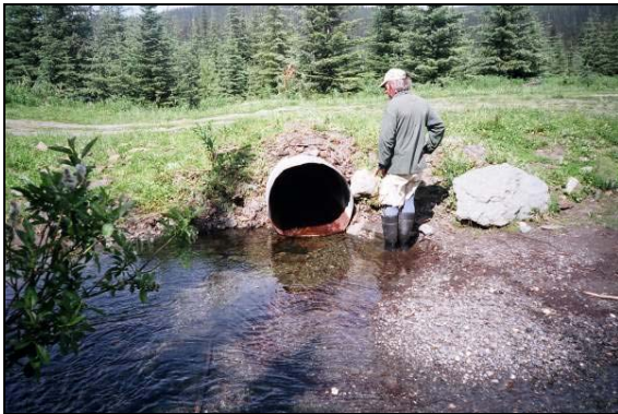
Photograph 2 – Site 13 Inlet Downstream View (Roll 1 10)
