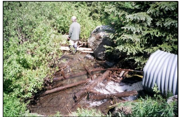
Photograph 4 – Site 13 Outlet Downstream View (Roll 1: 12)
