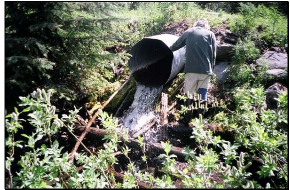
Photograph 3 – Site 13 Outlet Upstream View (Roll 1: 11)
