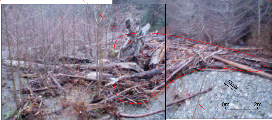
Photo 1: Downstream log jam at 0+500m
