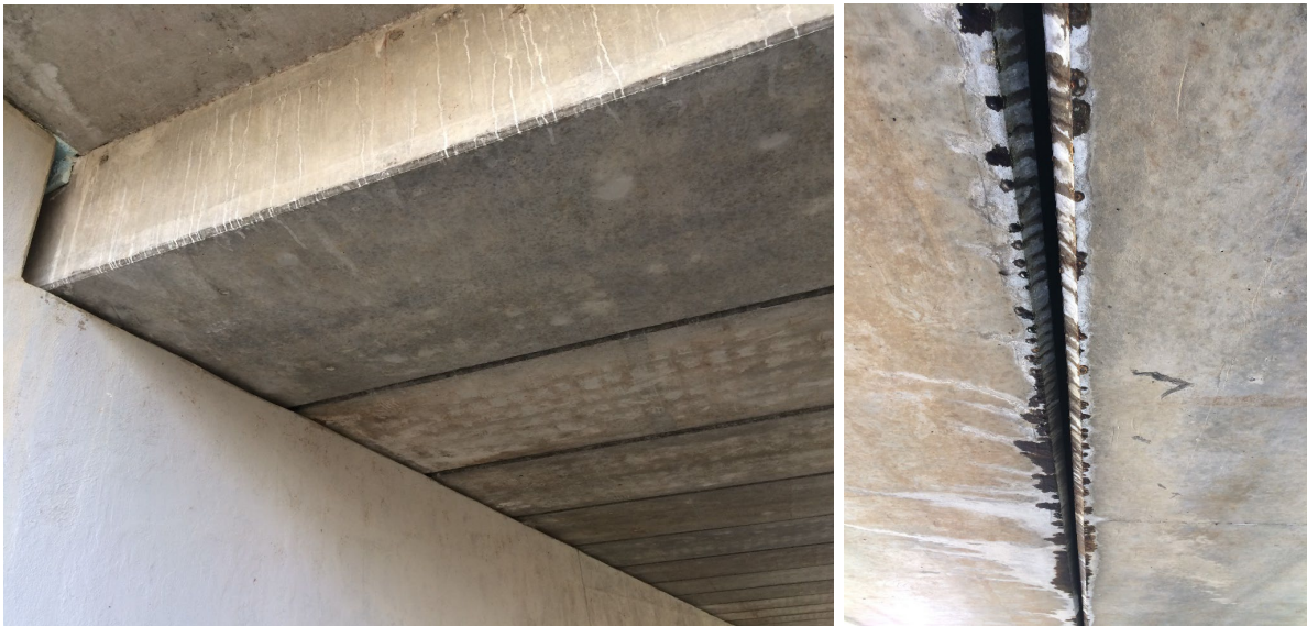
Figure 5. Expansion joints in a concrete bridge can provide roosting habitat (left). Staining around a joint may indicate use by bats (right). Photos courtesy of O. Dyer.
